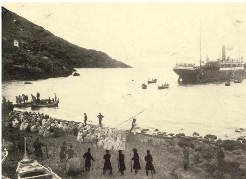
Figure 2. Arrival of Libyan deportees on Ustica, on board the steamship “Rumania”, 29 October 1911. The five guards in the foreground of the picture have been retouched by a pencil, under unknown circumstances. The Archive of the “Centro Studi Isola di Ustica” received the picture in this condition.
