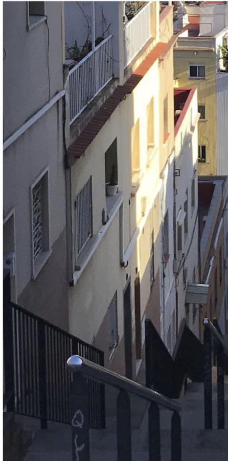
Figure 12. Dipòsit 10 in 2023 (authors).
