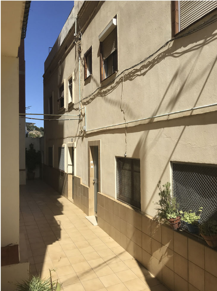
Figure 9. Pasteur 64, back building in 2022 (authors).
