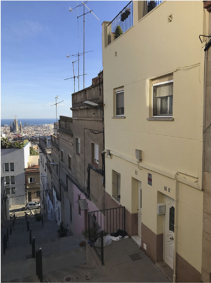
Figure 17. View of the building in 2023, more or less as in the 1955 plan (authors).
