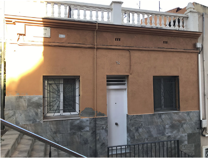
Figure 18. Passatge del Dipòsit 14, possibly also designed by F. Sanllehi Pont and barely modified, 2023 view (authors).
