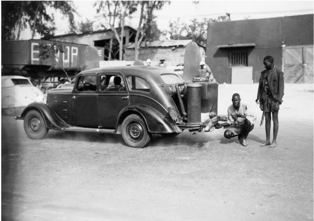
Fig. 2. Gazogène. Two men attending to a charcoal-powered engine in Senegal. Source: Photographer Unknown, Associated Press, 'Charcoal-Burning Automobile', 7 June 1942.
