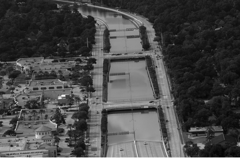
Figure 1.3 Interstate US-90 submerged in the aftermath of Hurricane Harvey, September 2017. Justin Sullivan/Getty Images.
