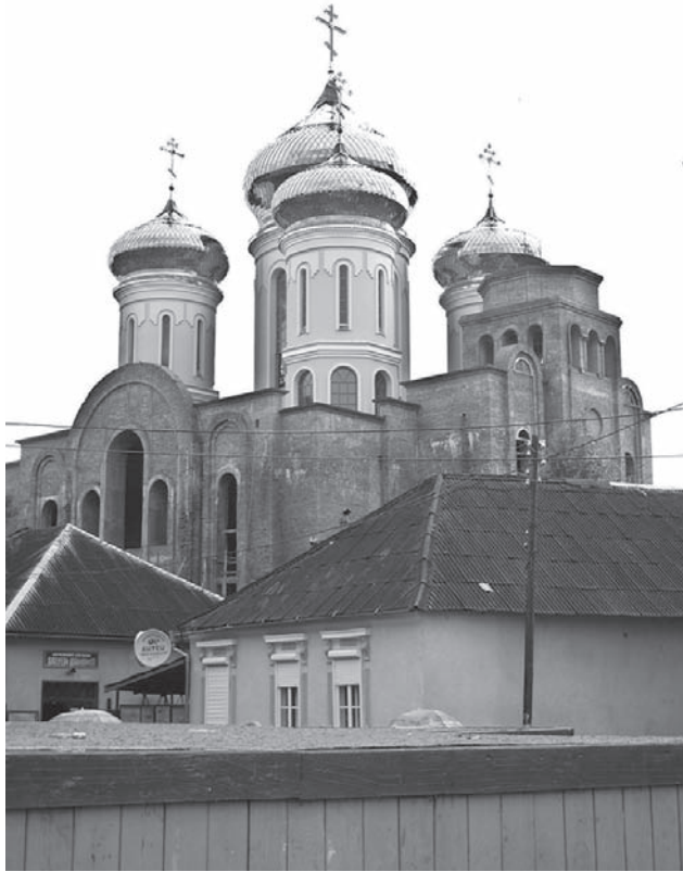
Figure 7. Hust (Ukraine), colossal Orthodox church in construction in the town centre, just behind the small traditional houses (Photo: Pál Lővei).
