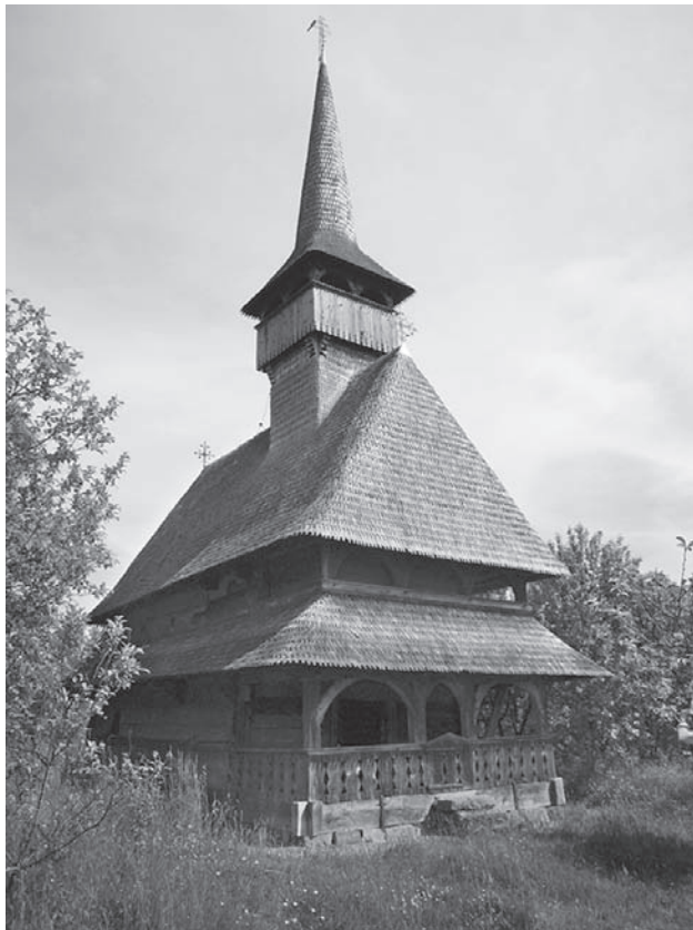
Figure 5. Bârsana (Romania), Romanian Orthodox wooden church, 18th century (World Heritage site) (Photo: Pál Lóvei).
