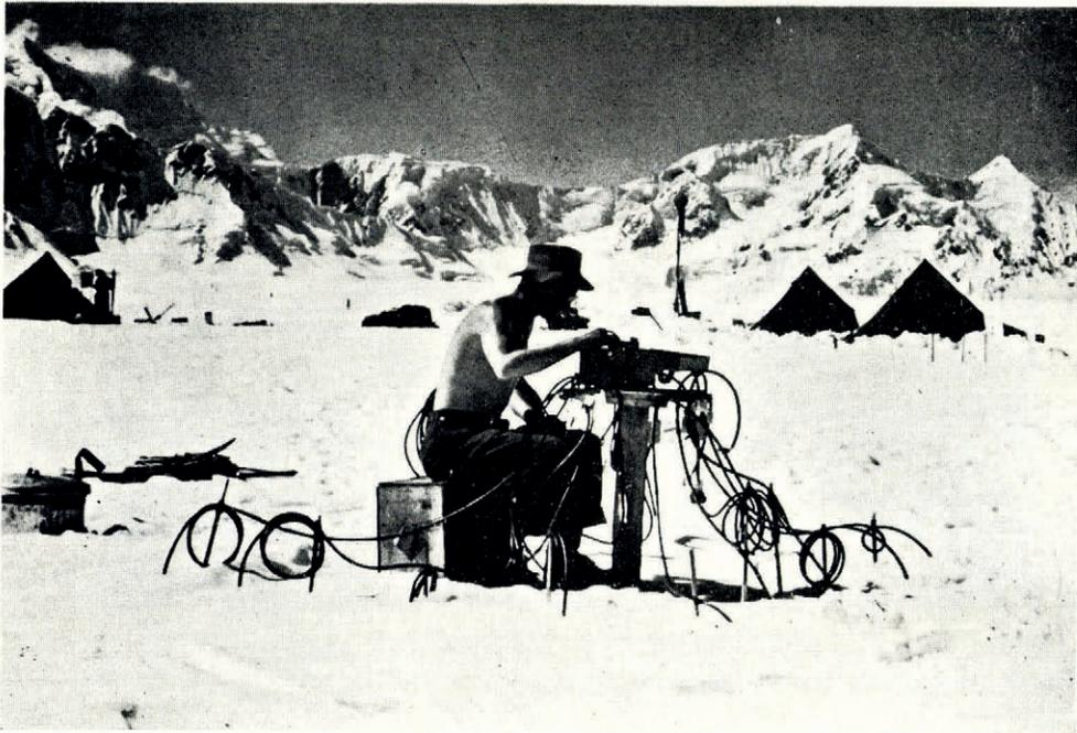
*Fig. 3. Temperature-measuring equipment as installed at Airstrip Station on the upper Seward Glacier (see text, p. 479)*
