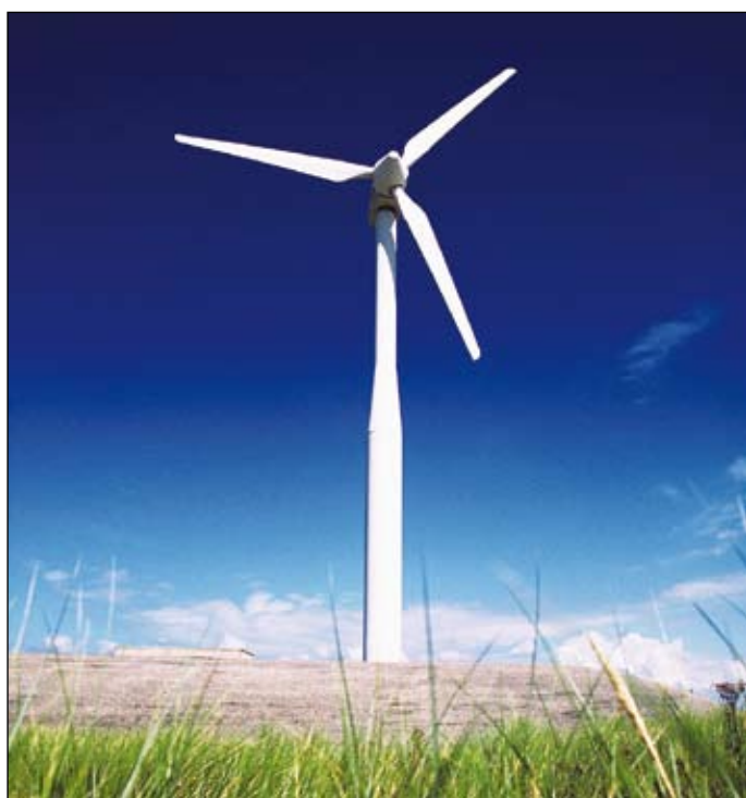
Wind turbines, a rapidly growing market. Source: World Steel Association
