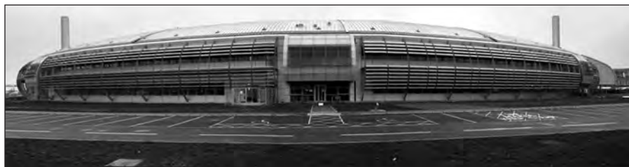
The Diamond Light Source, under construction in the United Kingdom. Photo taken in January 2006. (Photo: Diamond Light Source Ltd.)
