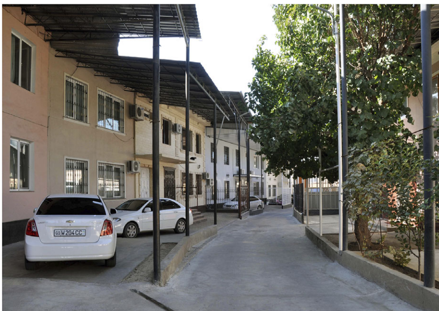
Figure 5. Housing in district C-27, Tashkent, Uzbekistan, 1973. Design by S. Adylov, I. Koptelova, and G. Korobovtsev. Author's photo, 2023.
