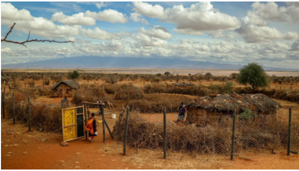
PLATE 1 A predator-proof boma under construction by the Born Free Foundation's Pride of Amboseli programme in 2018 ( Acacia thorn bushes have not yet been added to the outside perimeter).
