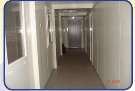
Inside MSF Hospital in Hattian Bala
