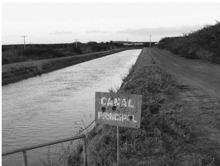
Figure 8. The main water canal which is an important infrastructure of an irrigation scheme. This publically built canal is located in the lower-middle-SFR in the municipality of Petrolina, Pernambuco, Brazil.
