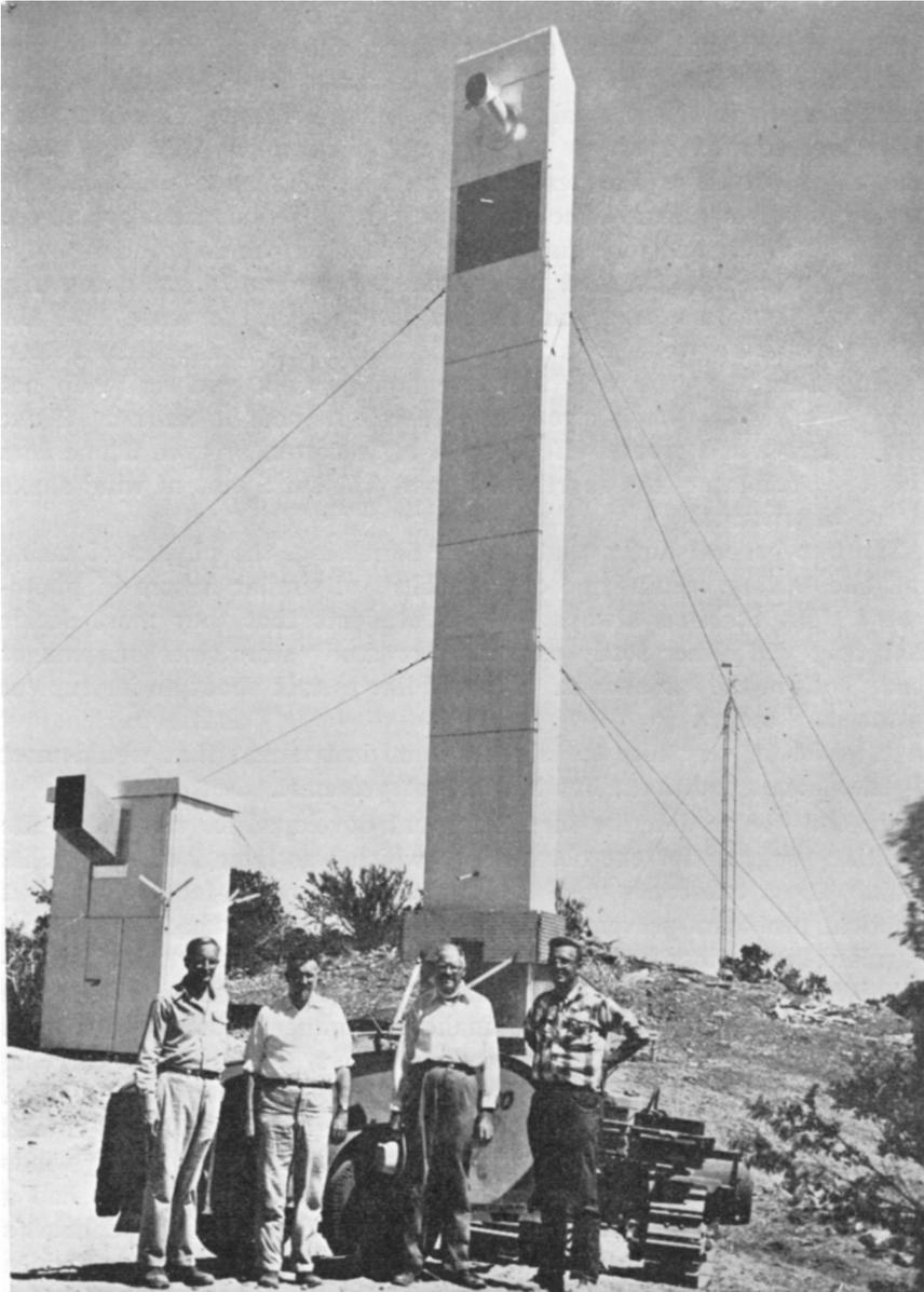
**Fig. 42.** — Photograph of the seeing test towers located on Kitt Peak. Polaris monitor telescopes are located in both the 10-foot and 60-foot towers. Microthermal probes project out the north face of 60-foot tower near the top and bottom. Note the outriggers supporting the outer tower shell. Shown are Drs. E. F. Carpenter, F. K. Edmondson, J. C. Duncan and A. B. Meinel.
