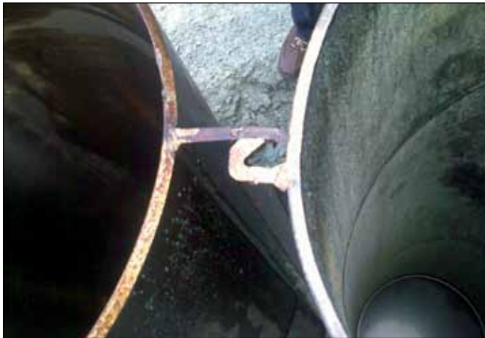
Ruukki's RD pile wall used in building a Road tunnel under a city in roadE6, Norway. Photo courtesy of Ruukki
