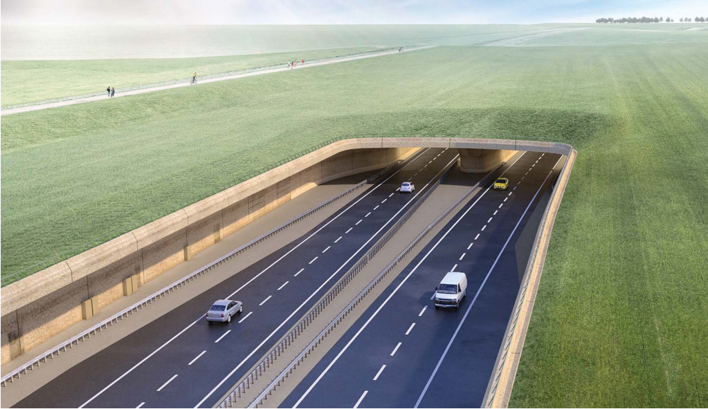
Figure 2. Proposed A303 tunnel western portal approach, with the existing road (top left) converted to a public right of way for walkers, cyclists and equestrians (© Highways England).
