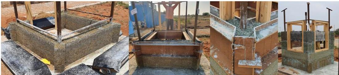
Figure 8: Photographs showing the layered casting of the wall
