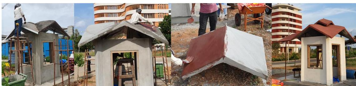
Figure 12: Finishing of the roof with cement plaster and cement punning
