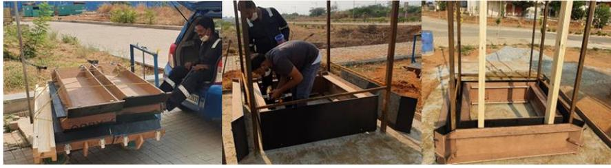
Figure 6: Transporting and installing the formwork at the site
