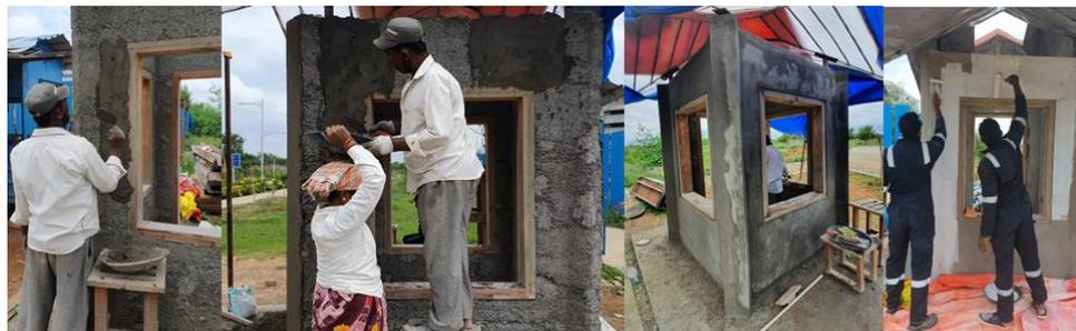
Figure 11: Plastering process of the Bio-Bricks wall
