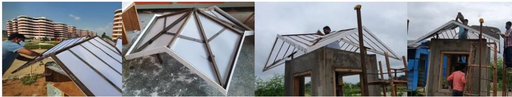
Figure 10: Fixing of the roof frame and casting of the roof
