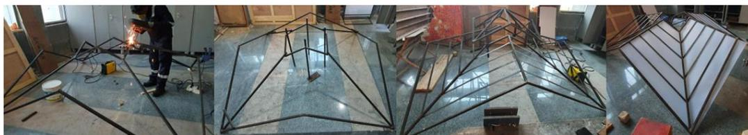
Figure 9: Making of the roof frame
