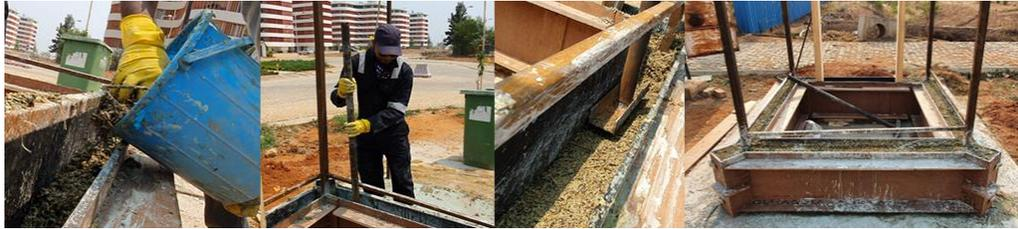
Figure 7: Pouring of Bio-Brick material, rans ramming and completion of the first layer
