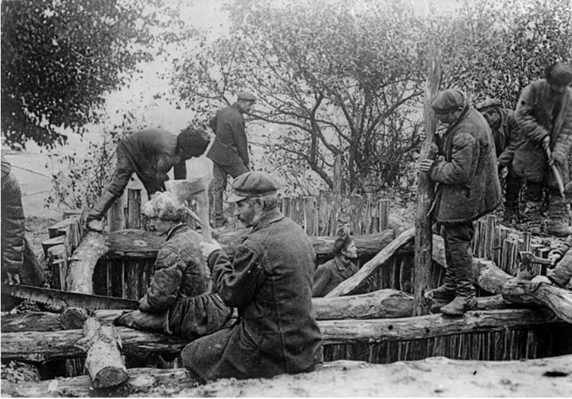
Figure 4. Construction of an Ice Cellar at an Agricultural Commune. RGAKFD I-7323 ch/b. http://photo.rgakfd.ru/photo/422444 .
