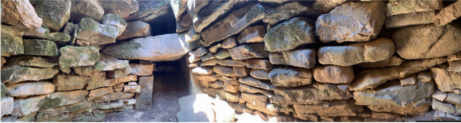
Fig. 3.17. CAPS: view of the inside of Tholos 14. © CIG.
