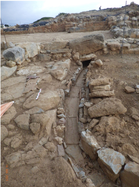
Fig. 3.72. Sissi: stone and terracotta drain coming from the Central Court in Space 6.12, seen from the east. © EBSA, J. Driessen.
