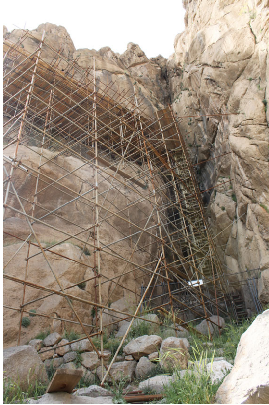
Fig. 2. Western wall of the gully at Mount Bisotūn, with the monument obscured by the scaffold (photo by the author)
