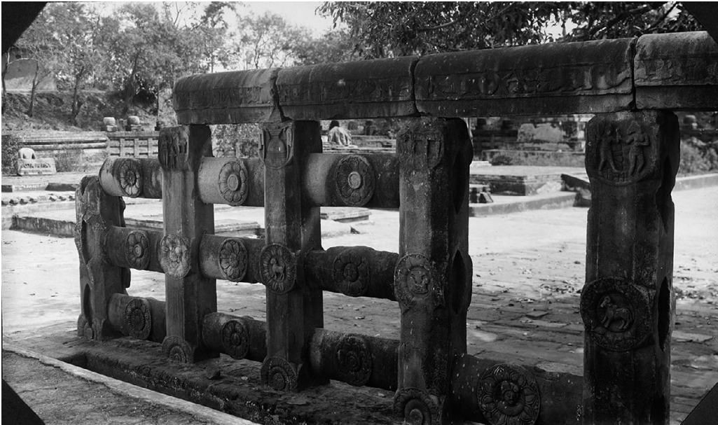
Figure 10. Stone railing at Bodhi Gaya, Bihar, India, constructed in a manner similar to wooden railings. From the Marshall photograph collection, held at the Oriental Museum, Durham University (Volume 41, # 3234).
