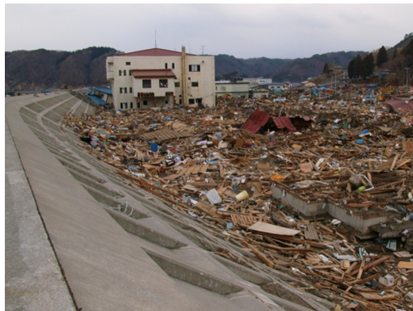
Figure 4. Tarō in the wake of the March 11, 2011 disaster. The great seawall was not tall enough to hold back the tsunami. Source (accessed 5-13-2011)
