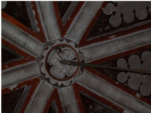
Fig 11. The octopartite rib vault in the vestiarium of Canterbury Cathedral. Photograph: © author
