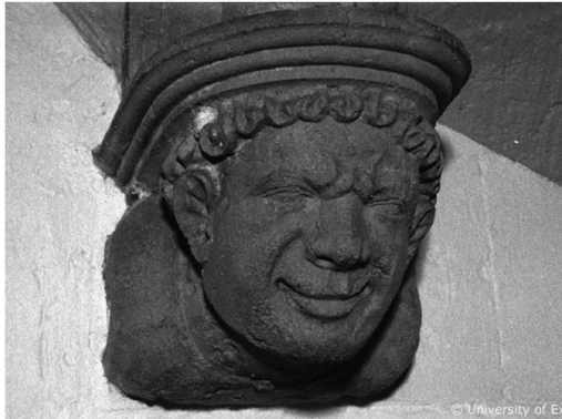
Fig 19. Exeter Cathedral: an example of a corbel supporting the vault ribs in the upper chamber of the northern treasure house. Photograph: © Exeter University
