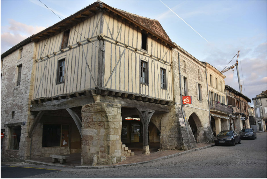
Figure 11. Villeréal, New Aquitaine, corner of Place de la Halle and Rue Saint-Roch, an example of structural and functional independence of the arcade and the room above.
