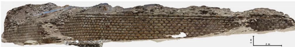
Figure 4. Orthophoto of revetment wall 2 in the northern sector of Tumshukayko A. On the left side, revetment wall 1 stands immediately in front of wall 2, partially covering the façade. (Color online)
