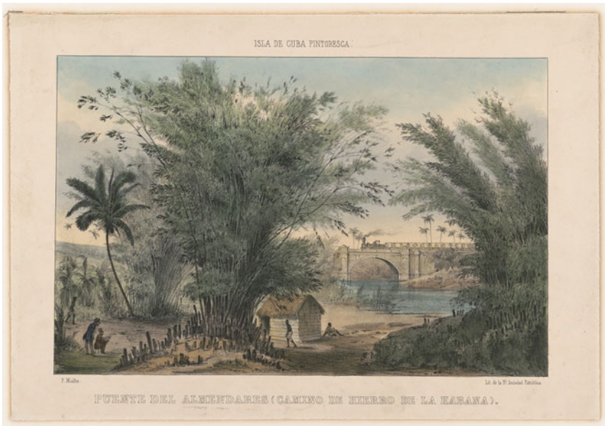
Figure 2. Railroad Bridge over the Almendares River near Havana. Library of Congress Prints and Photographs Division, Washington D.C., USA.
