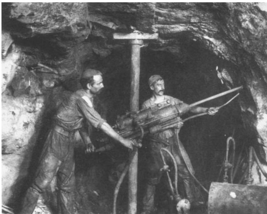
Figure 1. Cornish miners using a rock drill at the Carn Brea tin mine; ca 1900. The rock drill was dubbed the “widowmaker” by the miners, who recognized the deleterious health effects of increased dust from its use.
