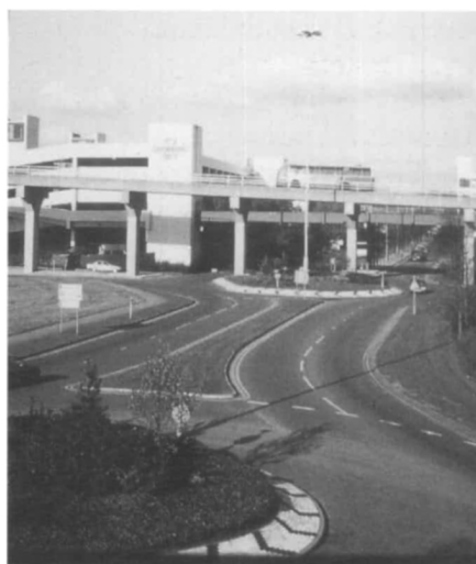
Fig. 8. Shopping City, Runcorn New Town, Runcorn Development Corporation, opened 1972. Vehicular traffic enters at ground level, pedestrians have their own walkways and buses have a third, elevated, access system
