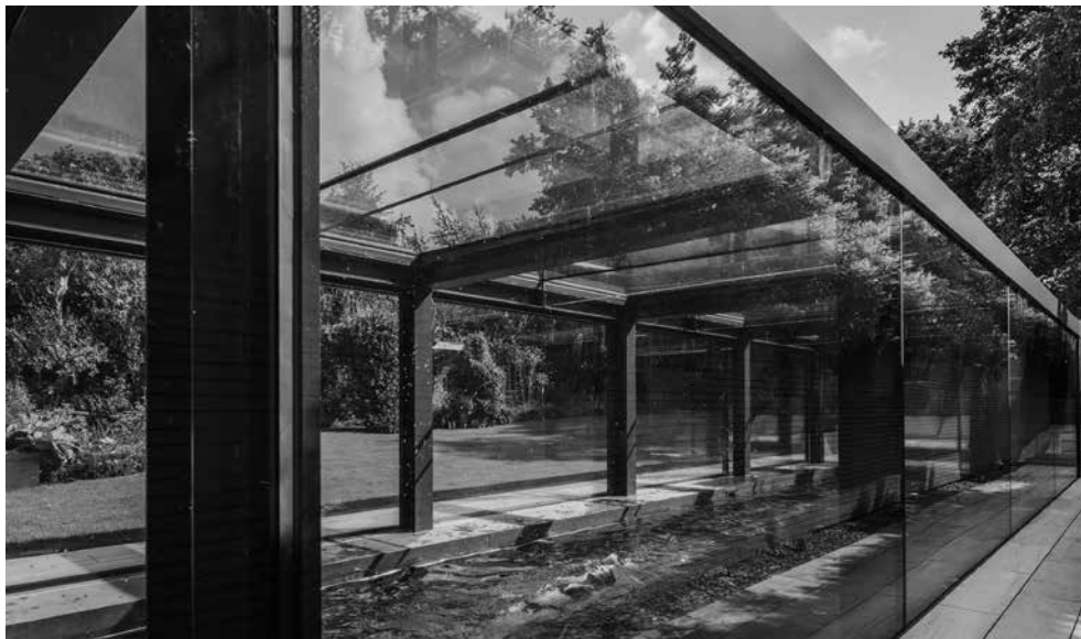
14 The glass enclosure showing transparency throughout.
