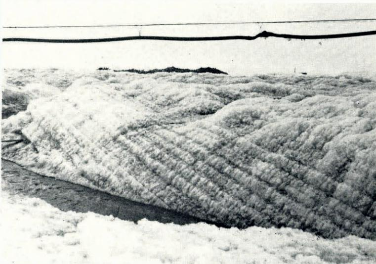
Fig. 6. Stratified ice at site III with strata 20 to 25 cm. thick
