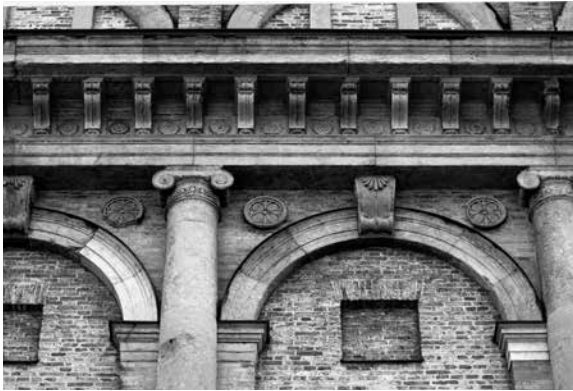
13 Hans Döllgast, detail of south elevation of Alte Pinakothek art gallery in Munich, reconstructed by Döllgast in the 1950s.
