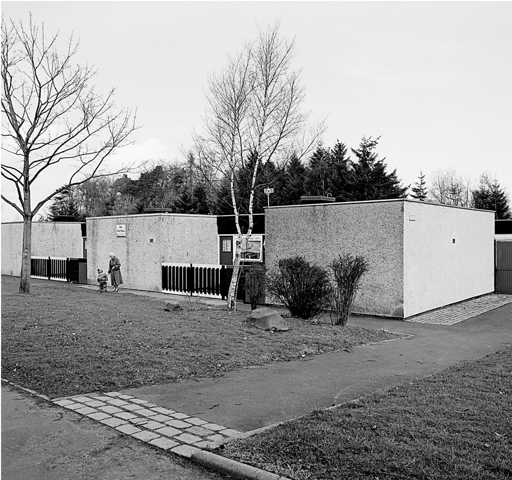
Fig. 16. Dundee, courtyard house on the Ardler estate, photograph of c. 1989 (Historic Environment Scotland)
