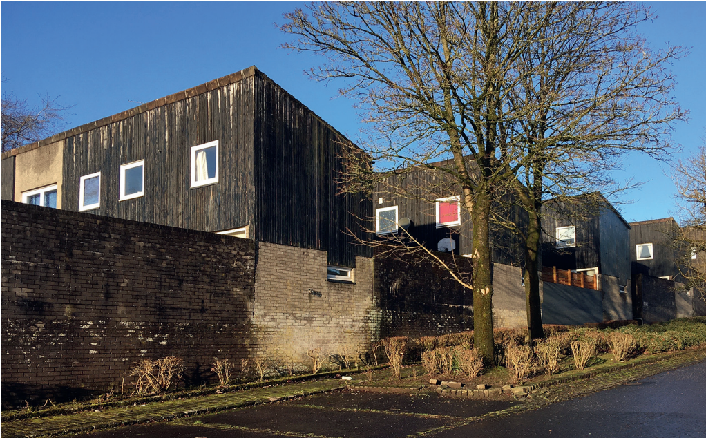
Fig. 10. Cumbernauld, single-aspect housing at Park 3 West (Maclehose Road), designed 1963–64 and built 1967–70, photograph of 2022 by the author
