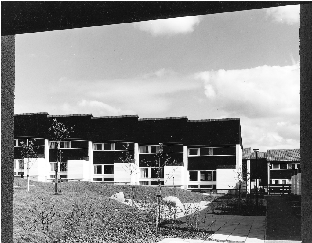
Fig. 5. Irvine, terraced housing by the Development Corporation at Pennyburn 2 with landscaped square, c. 1971 (Architectural Press Archive/RIBA Collections)
