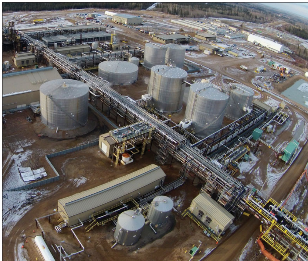
In situ bitumen recovery at the Surrmont oil sands project in northern Alberta. Credit: ConocoPhillips (November 2014).
