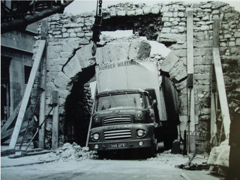
**Figure 2** Aftermath of collision, May 1964. South-facing aspect of Newport Gate, with lorry jammed between it and the ground surface. Photo courtesy of Lincoln Central Library and Lincolnshire Archives, reference LCL 26000.
