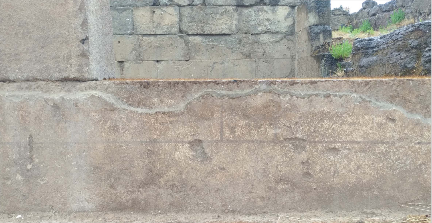
Figure 6. Painted plaster on the interior of the Area F complex mimics the worked local stone used to construct the building (figure by the Gabii Project).
