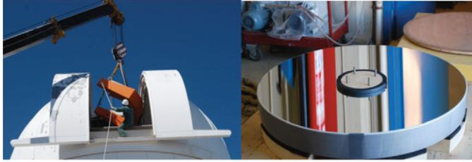
**Figure 2.** (left) Dismantling of the MARLY telescope and (right) aluminizing of the primary mirror.
