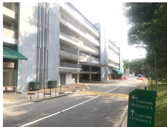
Multi-story Carpark (MCSF).
