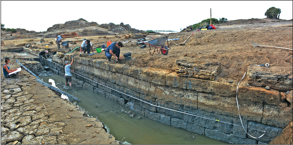
Figure 3. The southern wall of the 'Kothon', section M.4575 (see Figure 4), separating the pool from the Marsala Lagoon; viewed from the north (© Sapienza University of Rome Expedition to Motya).
