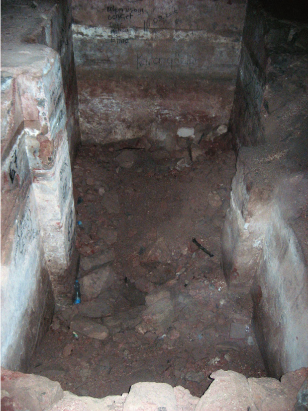
Figure 7. Cistern (photo by author, 2012).
