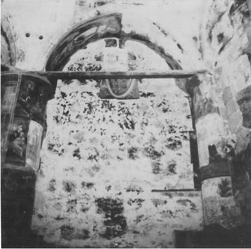
Wall of a looted church in northern Cyprus, photographed by Robin Cormack during his study-tour. The rough squares on the wall mark the large area where a complete Last Judgement has been removed, patch by patch, leaving only two fragments in the upper part of the wall. More paintings have gone from the column on the right, and some from that on the left. (Reproduced with the permission of the Council of Europe.)
