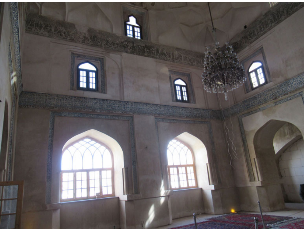
Figure 4. Dome chamber, northeast view
