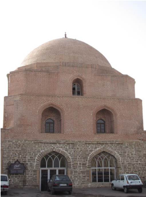
Figure 5. Dome chamber, north façade
