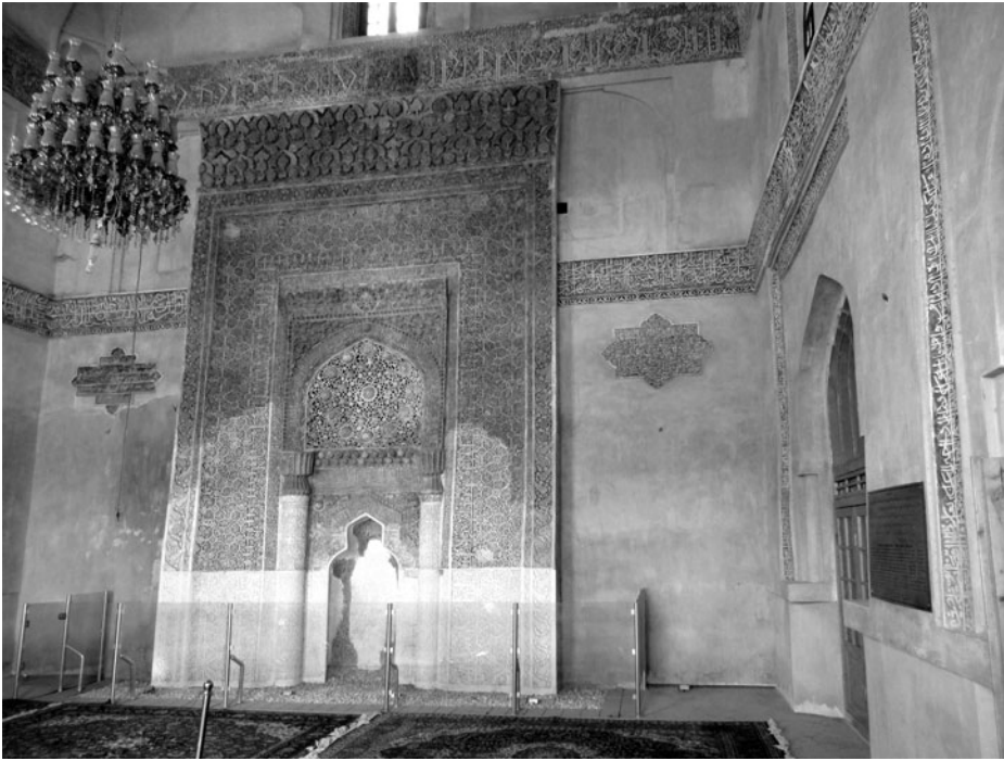
Figure 9. Dome chamber, view of the mihrāb and qibla wall
