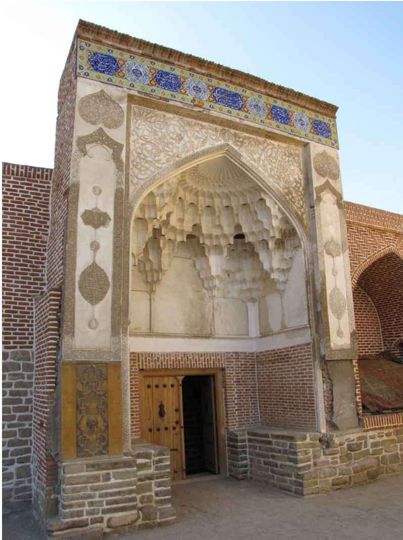
Figure 17. View of the west shabistān portal
