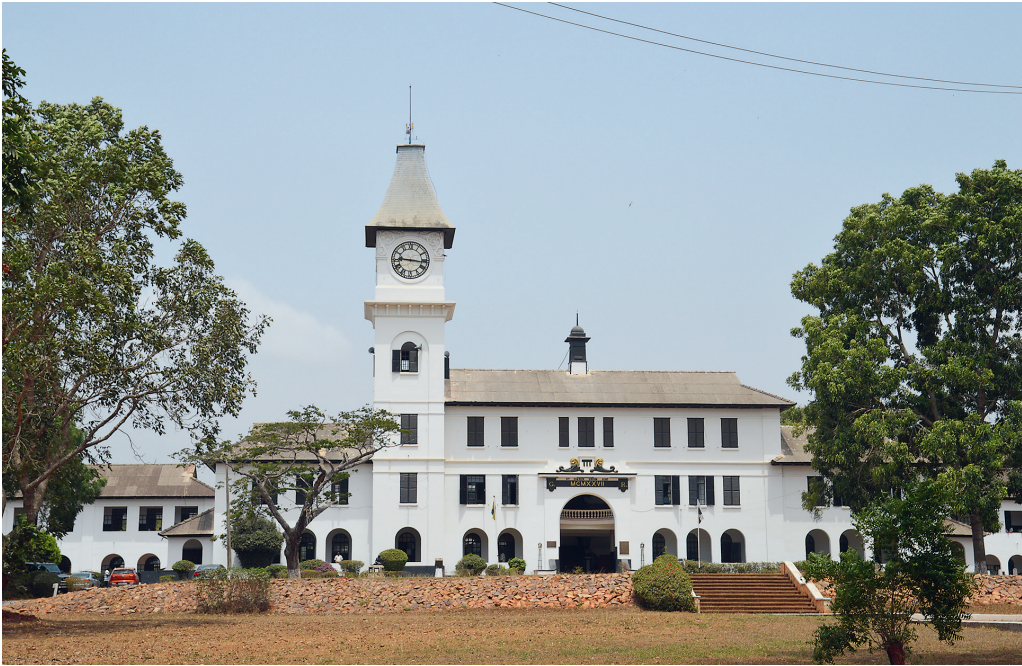
Fig. 1. Achimota School, Accra, by Walter Frederick Hedges, 1920, photograph of 2019 by the author
