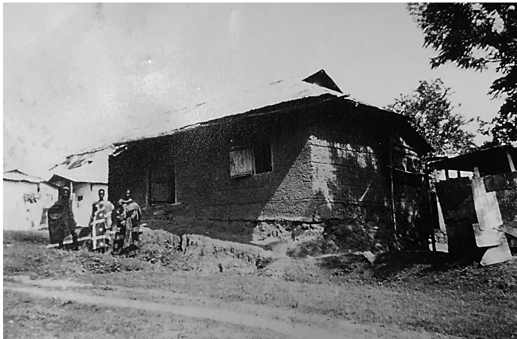
Fig. 2. Alcock's experimental 'swishcrete' housing in Kumasi, photograph of 1944 (private collection)
