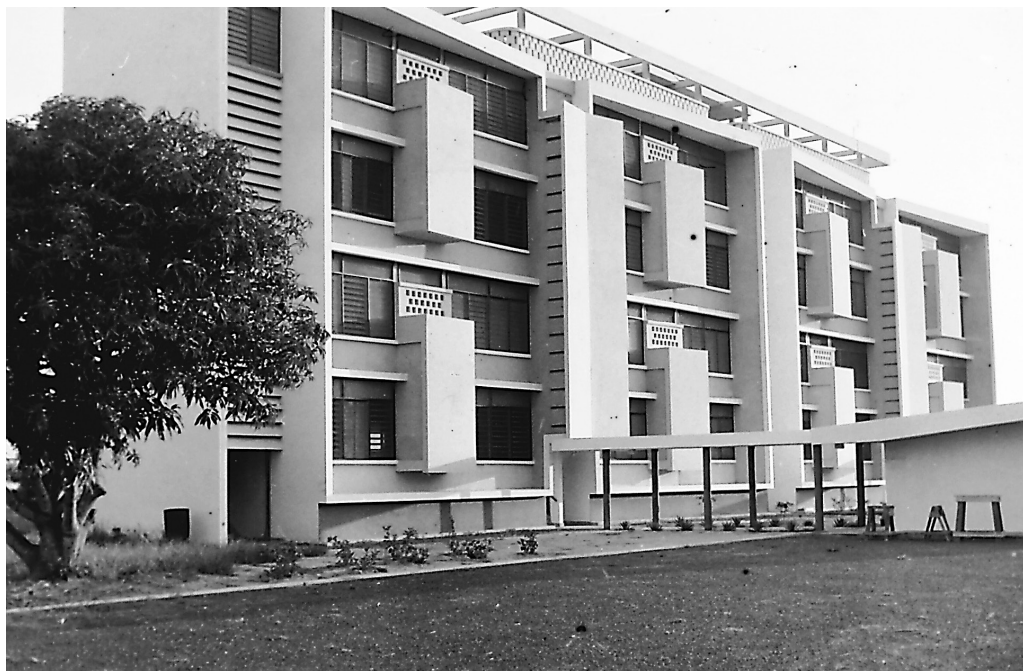
Fig. 8. Tema Community 1, maisonettes by Drake and Lasdun, 1957, photograph of 1957 by Michael Hirst
