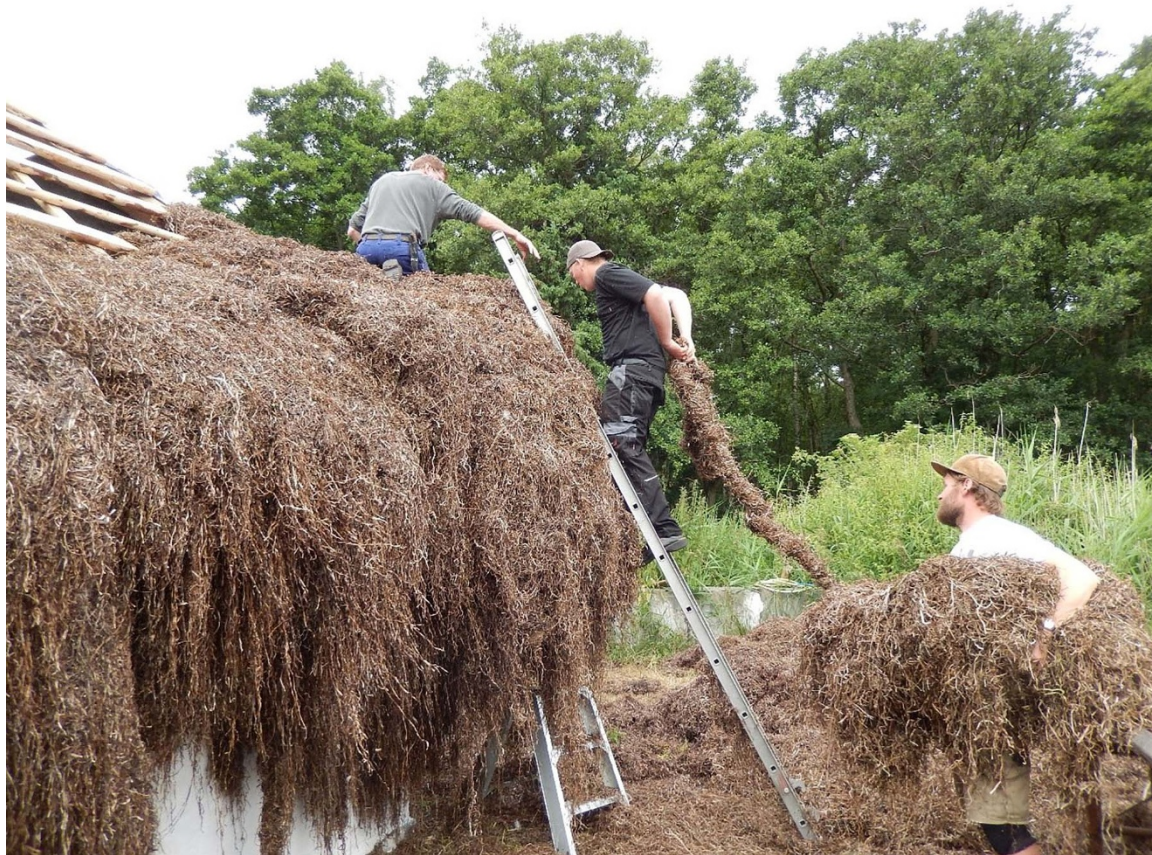
Figure 2. Example of a seagrass thatched roof on a Danish House © visitlæsø.
