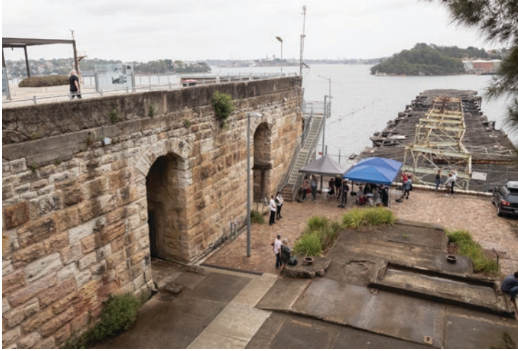
Figure 2. A former coal loader facility with two tunnel entrances and a flight of stairs to access the rooftop abutment Sydney Harbour. People gather outside the facility next to rusted scaffolding of the former loading dock. The Coal Loader Centre for Sustainability on Sydney Harbour, 2020. (Photo by Daniel Boud)
