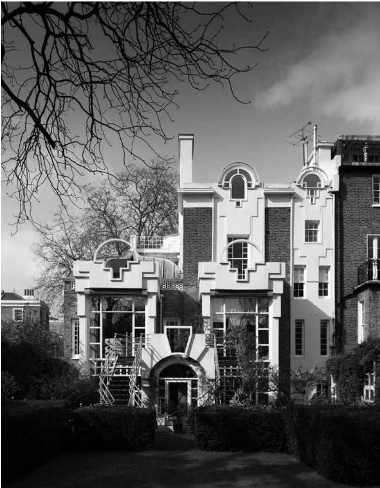
2 Thematic House, a.k.a. Elemental House, Cosmic House; 19 Lansdowne Walk, Kensington & Chelsea, Greater London. Charles Jencks with Terry Farrell, 1979–85. Rear elevation from south.
