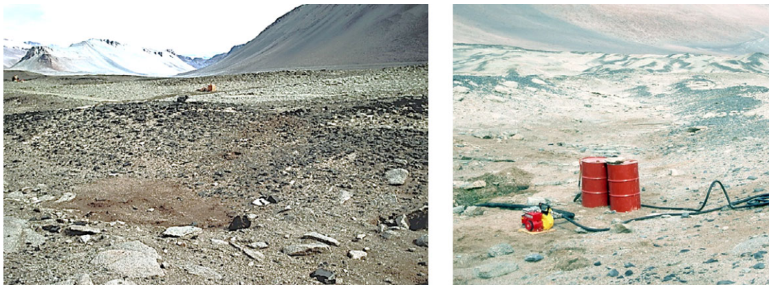
Figure 6. Greywater Gully, where liquid washing waste (personal and from kitchen) was deposited from 1969 to 1990. Left, the site prior to remediation in 1992; right, pump removing contaminated groundwater for transport back to Scott Base.
