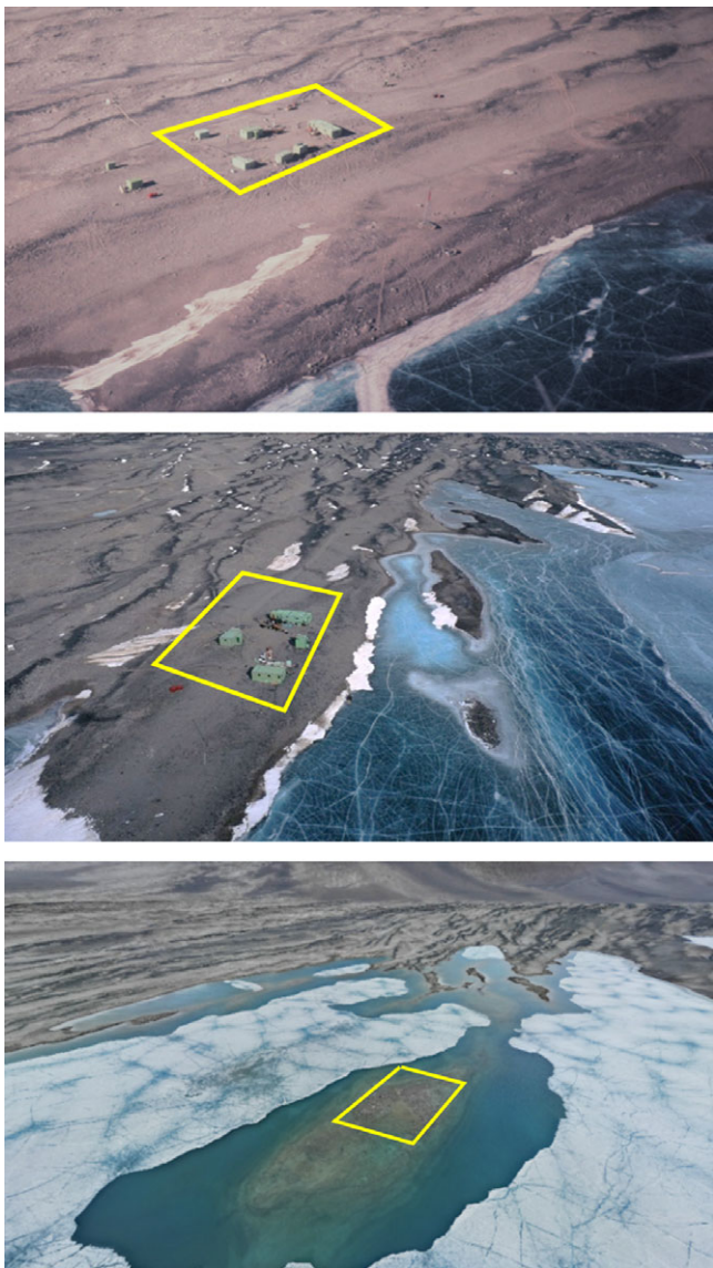
Figure 4. Vanda Station in the 1970s (top), at the time of removal in 1993 (centre) and the flooded site in 2023 (yellow boxes mark the same footprint of the station in all images).
