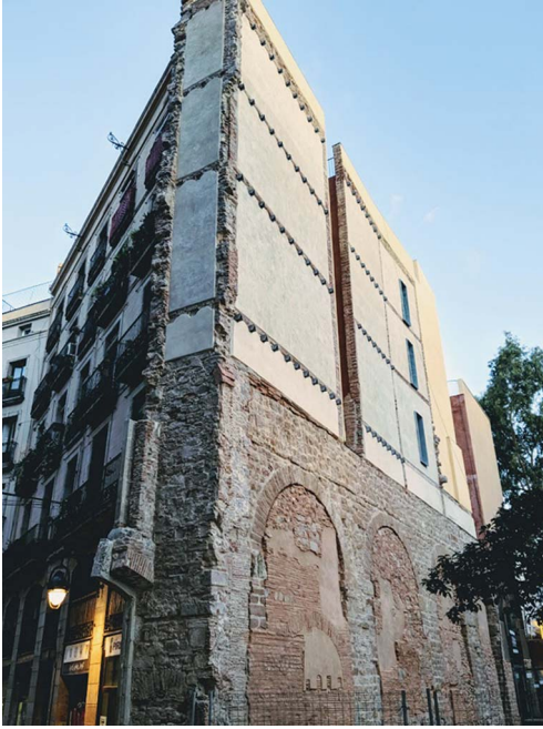
Figure 1. The newly displayed arches of Barcelona's Roman aqueduct preserved within the structure of a later building on the Carrer de Duran i Bas (photograph by R. Witcher).
