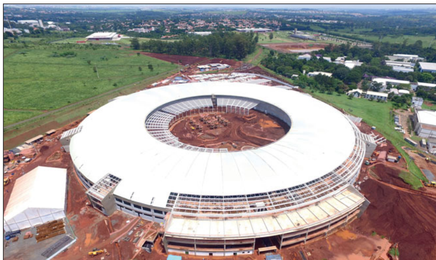
The construction site of Sirius, Brazil's new fourth-generation synchrotron light source. Sirius could greatly increase the capacity of Brazil's research infrastructure, but scientists are already struggling to maintain adequate support for existing research. Credit: LNLS/CNPEM.
