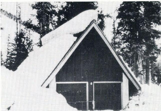
Fig. 7. Appearance of a tensile crack high on a roof caused by gliding. Equation (6) provides estimates of stresses on a barrier where  $X_0$  is shown in Fig. 6b.
