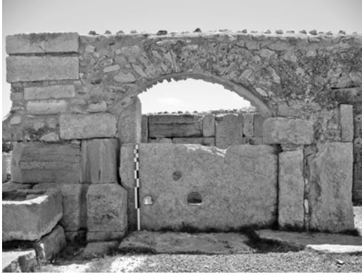
Fig. 8. Sbeitla: holes in the balustrade of the northern fountain. (Lamare 2017, fig. 15.)
